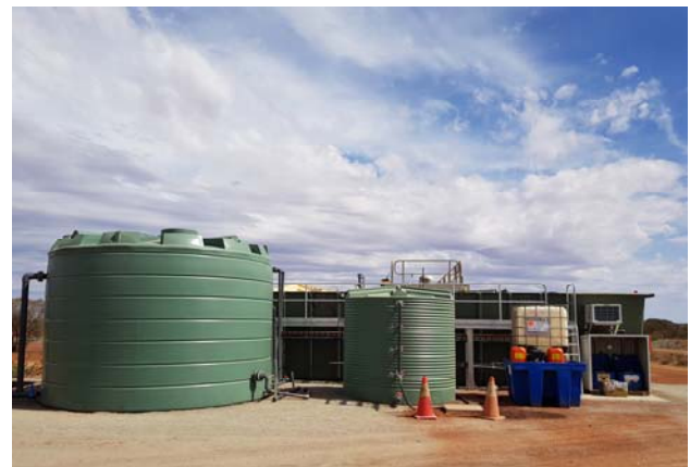
MAK Water modular ASBR plant installed onsite
