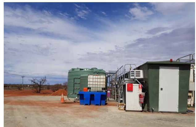
MAK Water ASBR plant with integral plant room
